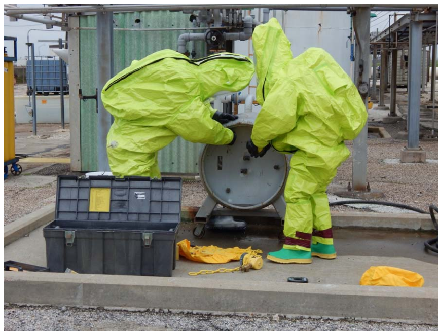
Figure 2. Live drill with HAZMAT team members installing a chlorine cylinder patch kit. Live drills provide the most realistic simulation of a real situation. [Color figure can be viewed in the online issue, which is available at wileyonlinelibrary.com .]
